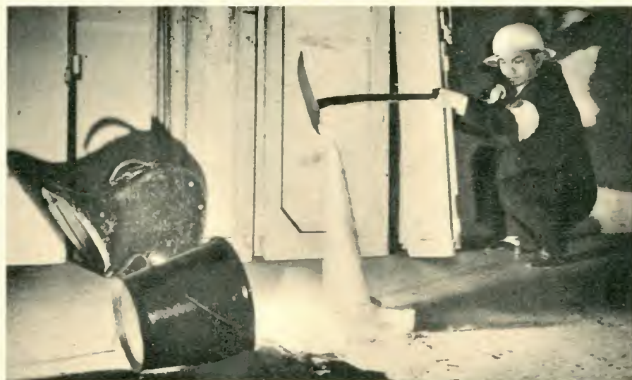
2. CONTINUE piling sand on the bomb to keep the sparks from flying. Your job is not to put the bomb out but to keep its fire from spreading. Keep at this job until the activity of the incendiary slackens
